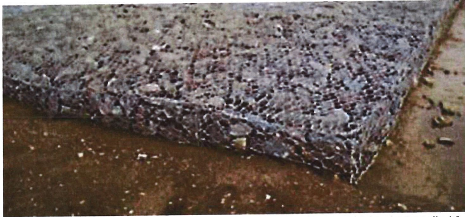
Figure 5. Rock-filled gabion mat, similar to the kind that is proposed to be installed for added protection of fibre optic cable from the cable vault, through the intertidal zone, to the mean low tide line.
