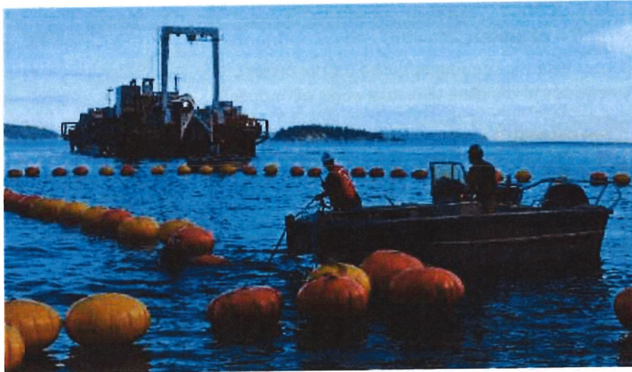
Figure 3. Cable being pulled ashore from cable laying vessel by a smaller boat. Floats are being attached to cable to prevent cable from sinking. Floats will later be cut by divers who will ensure cable is accurately placed within approved right-of-way.
